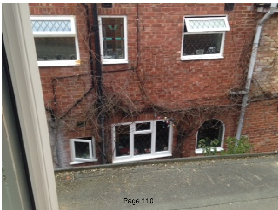
View towards no 25 with the casement window open
