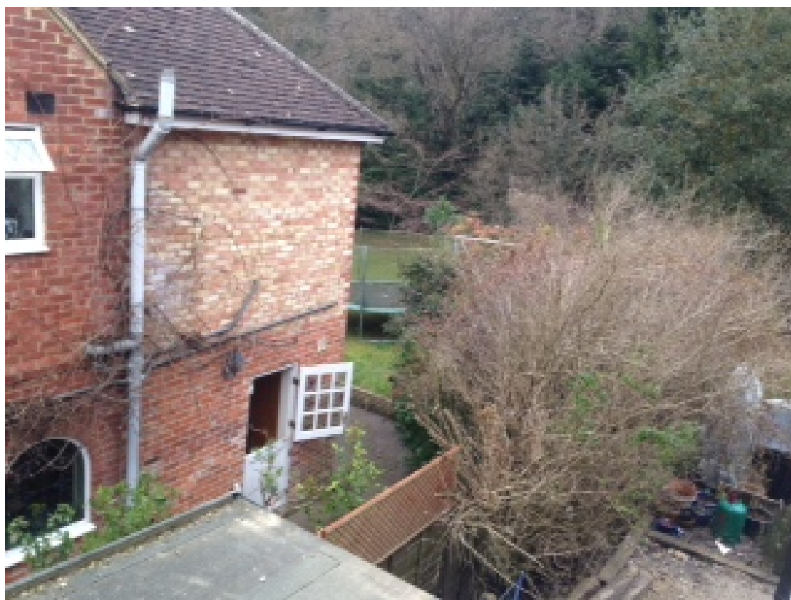
View towards the rear of nos.25 and 27 with the casement window open
